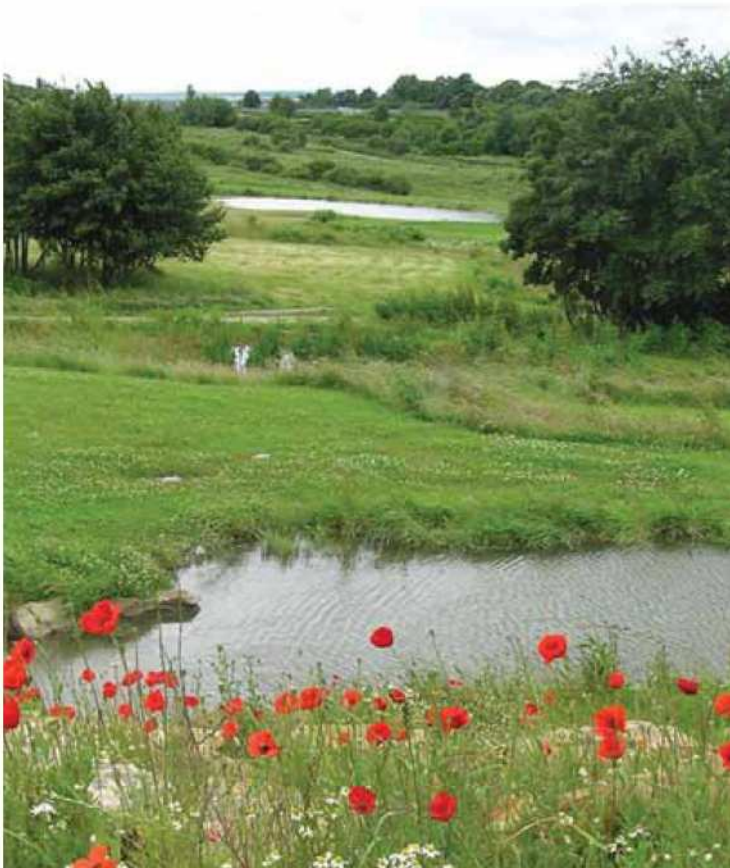
Figure Q: SuDS detention basins serving social housing developments on the Manor Estate in Sheffield
