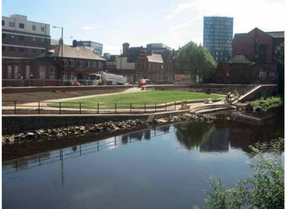
Figure G : Nursery Street, Sheffield – New flood defences and a pocket park built in 2012
